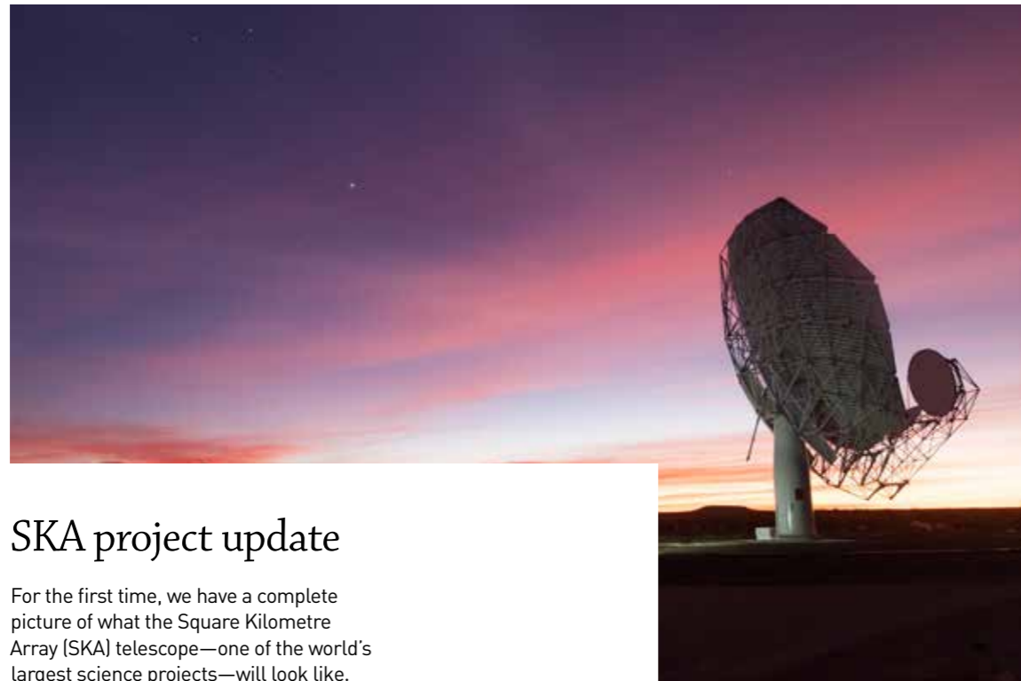
The MeerKAT radio telescope in South Africa is an SKA precursor consisting of 64 dish antennas each 13.5 metres in diameter. Credit: SKA South Africa.
